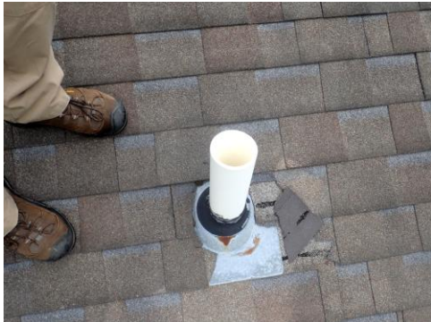
Plumbing boots leaking - The rubber neoprene boot has split and deteriorated due to age.
