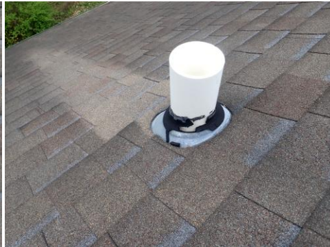
Plumbing boots leaking - The rubber neoprene boot has split and deteriorated due to age.
