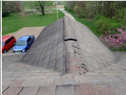
Cap shingles need updated ASAP or best would be just replace roof.
