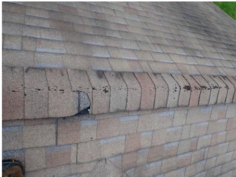
Cap shingles need updated ASAP or best would be just replace roof.
