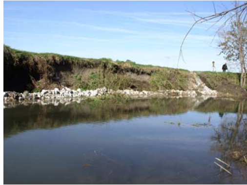
Stone Toe Protection
