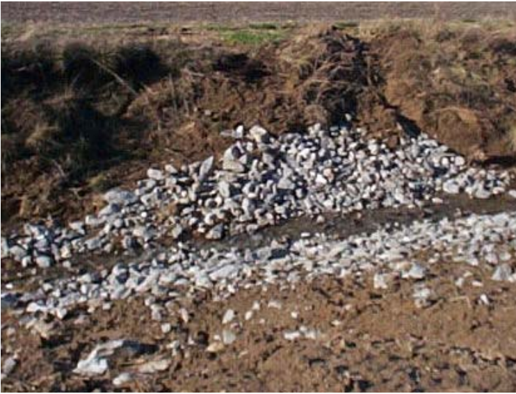
Streambank Stabilization Project using RR-4 Stone
