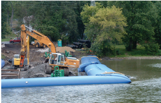
Aqua-Barriers in the Fox River at Batavia help assure an accessible construction site while protecting the river from construction site erosion.
